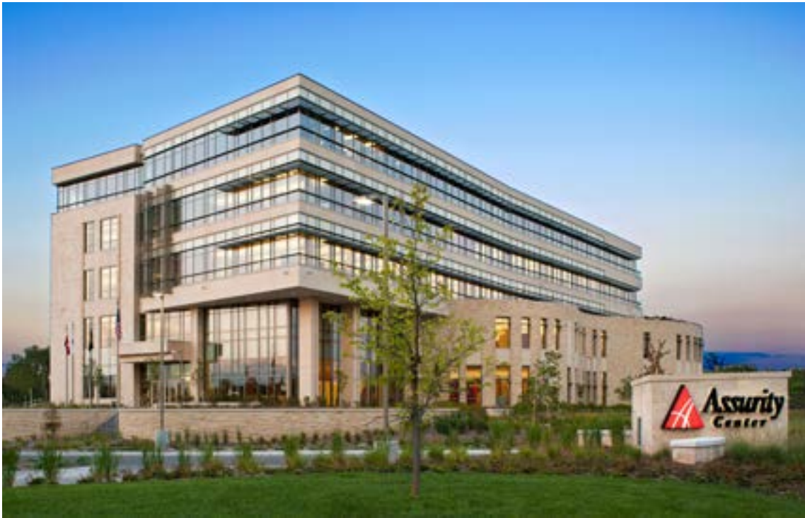
▲ The Assurity Center in Lincoln, Nebraska is a model for other companies looking for ways to ensure environmental sustainability. The Center has been designated as a Groundwater Guardian Green Site in recognition of its groundwater-friendly practices.
