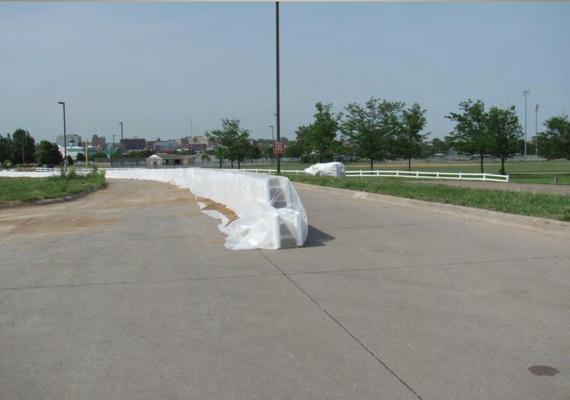
Temporary dike erected at South Sioux City
